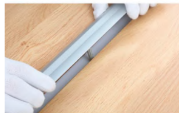
3. Position screws over hole
