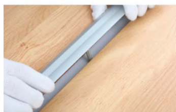
3. Position screws over hole
