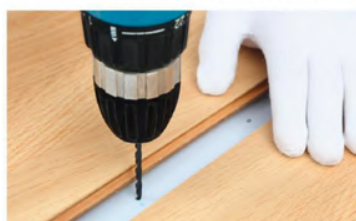
1. Hole positioning & drilling using 6mm drill bit
