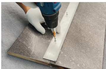
1. Hole positioning & drilling using 6mm drill bit
